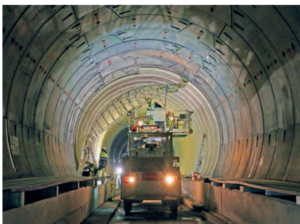
The composite plates are laid over the concrete segments forming the tunnel lining. They channel the incoming water through the sidewalls.
