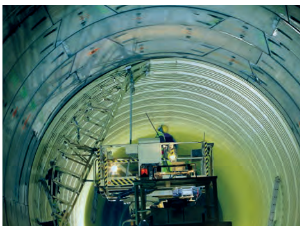
The composite plates are laid over the concrete segments forming the tunnel lining. They channel the incoming water through the sidewalls.
