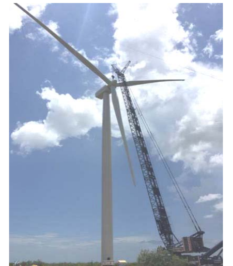
6. A rotor (blade assembly) is installed.
