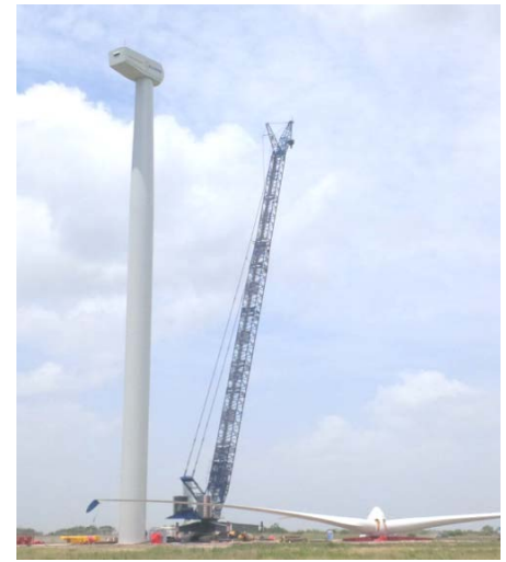
5. An erected nacelle ready for rotor installation
