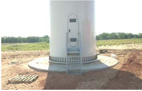
1. An installed tower base.
