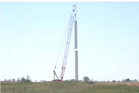
3. An upper mid tower section is installed.
