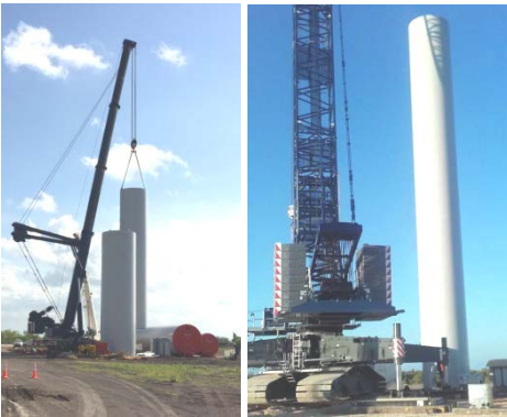
2. A lower mid tower section is installed
